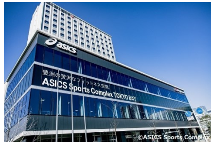
ASICS Sports Complex TOKYO BAY
